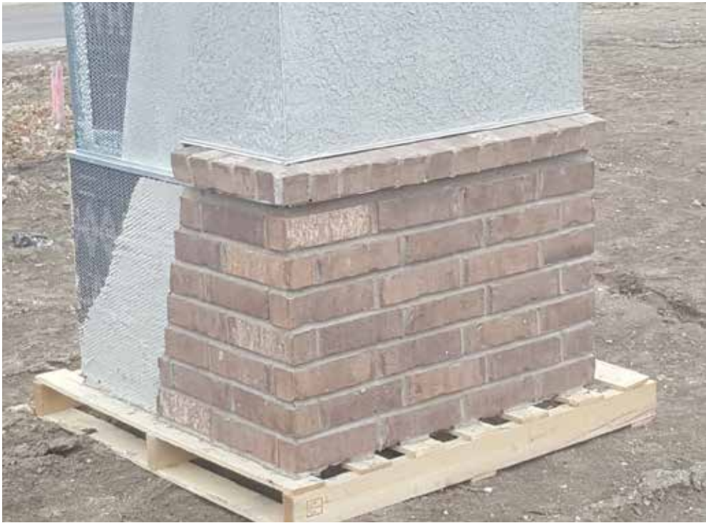
FIGURE 2.4 THIN BRICK APPLICATION GOOD EXAMPLE
