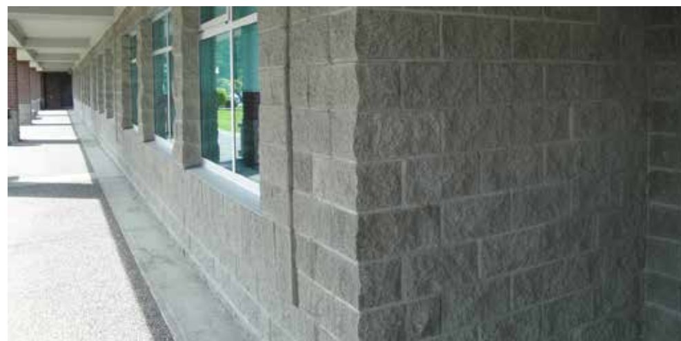
FIGURE 2.3 SPLIT-FACE BLOCK EXAMPLE
