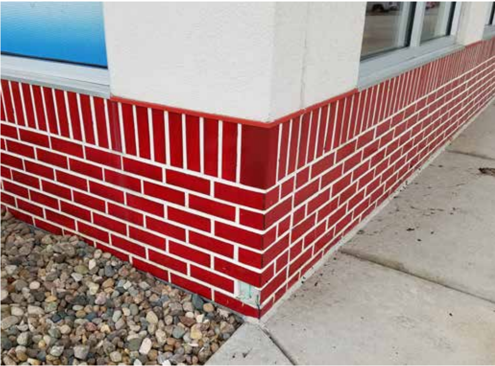
FIGURE 2.6 THIN BRICK APPLICATION BAD EXAMPLE
