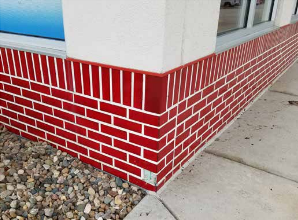
FIGURE 2.6 THIN BRICK APPLICATION BAD EXAMPLE
