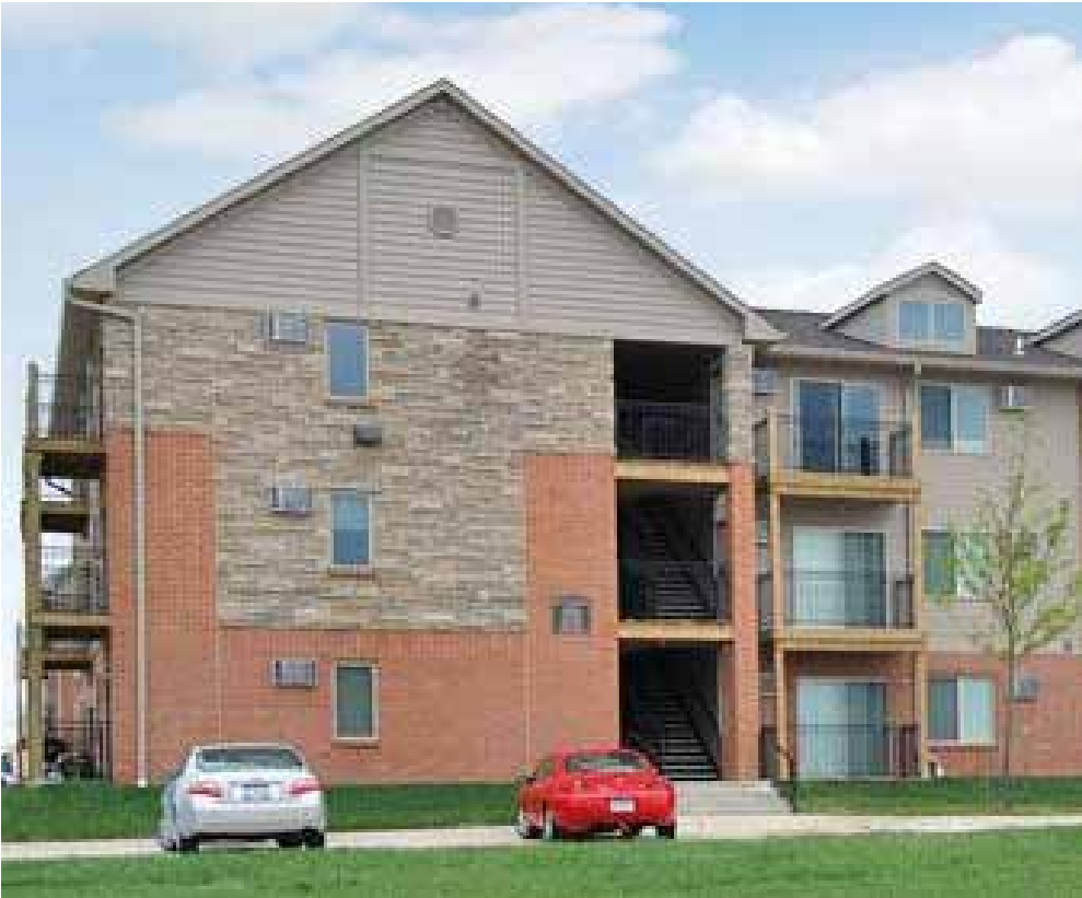
FIGURE 2.7 BUILDING WITH INSUFFICIENT TRIM
