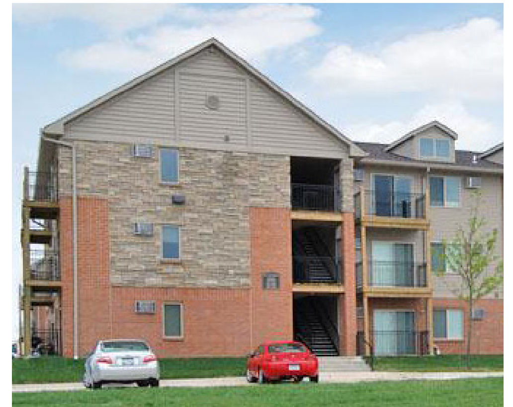
FIGURE 2.7 BUILDING WITH INSUFFICIENT TRIM
