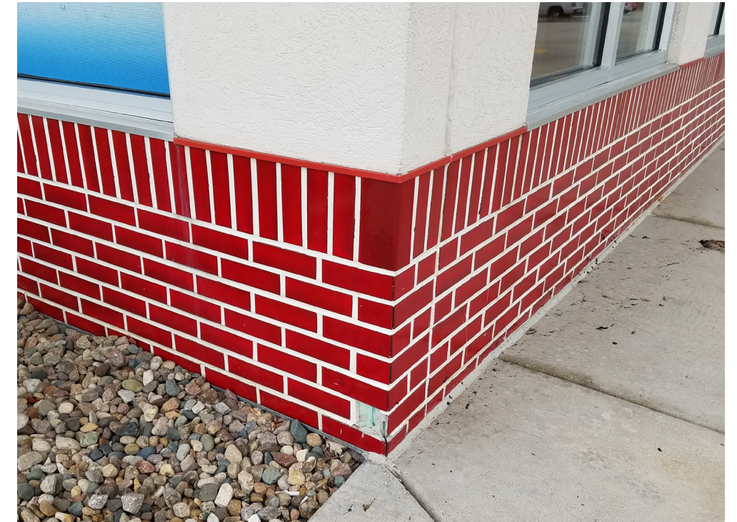
FIGURE 2.6 THIN BRICK APPLICATION BAD EXAMPLE
